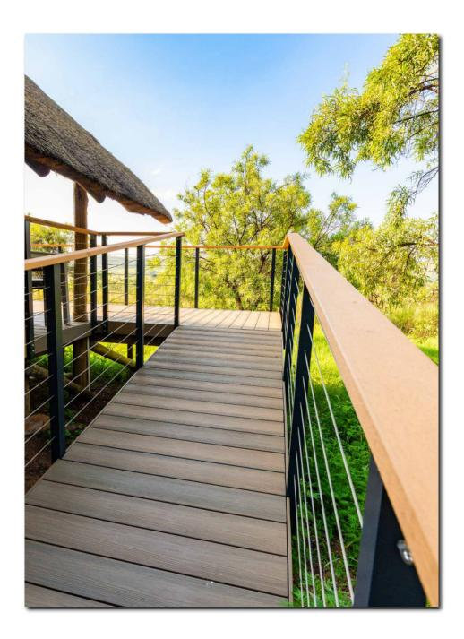
As one of the toughest co-extruded composites available, Infinity offers decay and weather resistant decking in convenient, lightweight I-series profiles. The smart-shaped channels of each board are deliberately designed to use less material while providing the dimensional strength and stability necessary for extended spans such as those at the pavilion and the restaurant deck.
